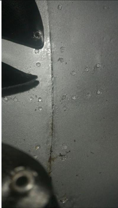
*Photo of dome showing no bead, any joins appear to be more the galvanized paint pooling rather than a weld*
